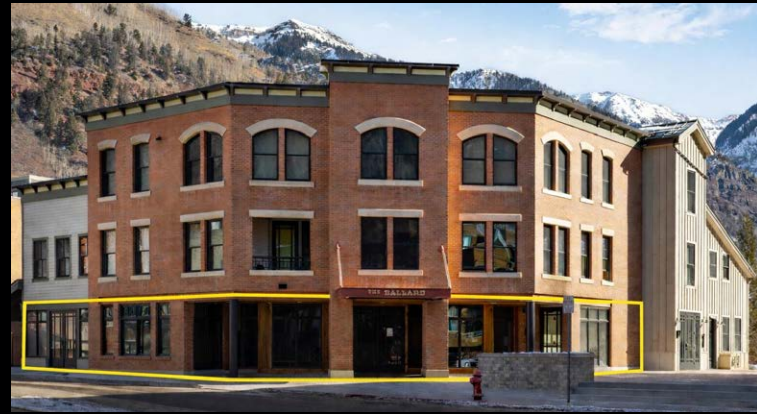
Ballard House North Units CR-101 & 102 // $5,275,000
